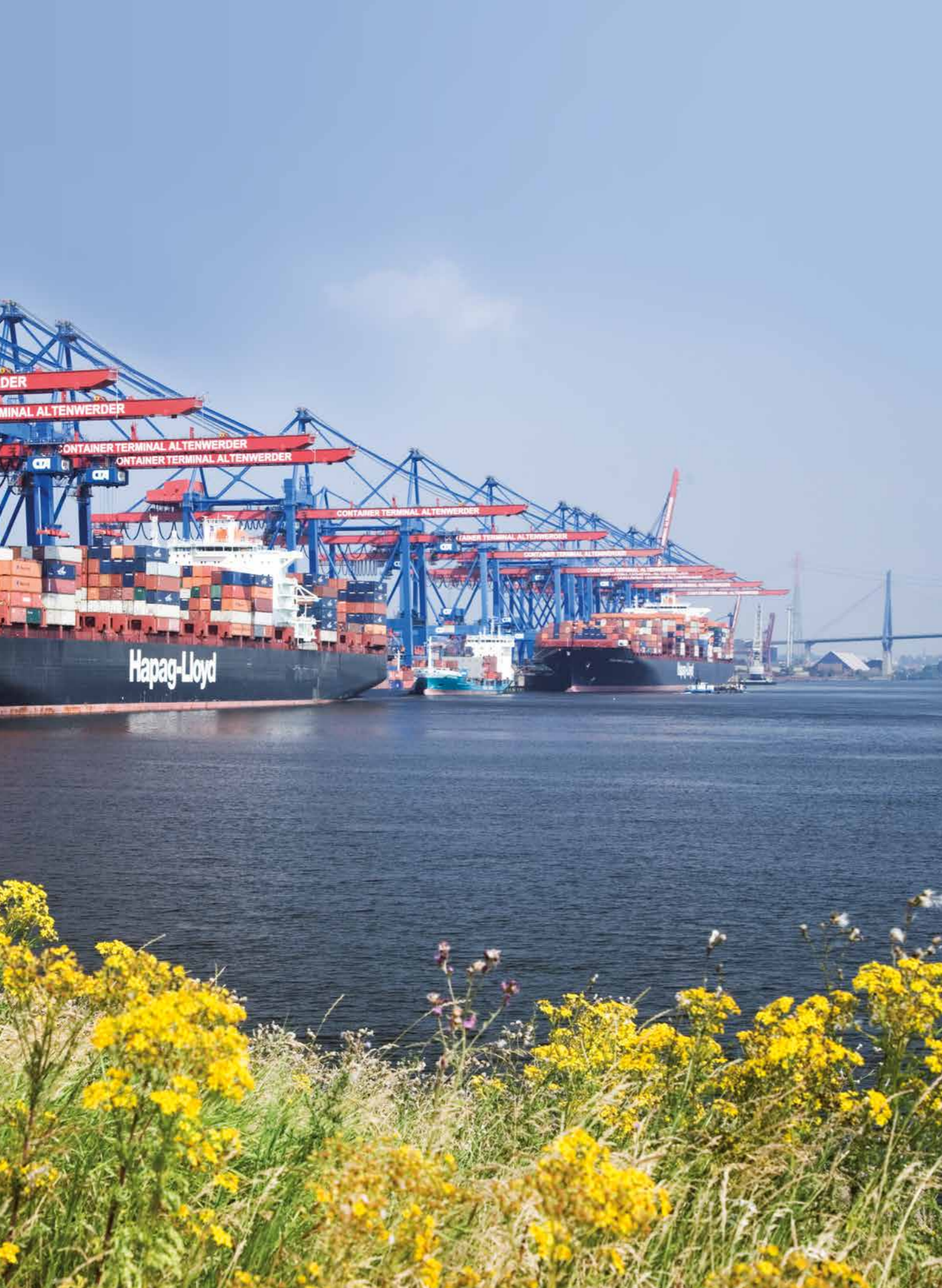
The Ballin Quay in the HHLA Container Terminal Altenwerder, Hamburg
