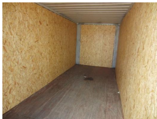
Figure 7.53 Lining a 40-foot container with chipboard panels
