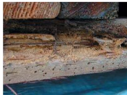
Figure 6.13 Wood frass from boring insect
