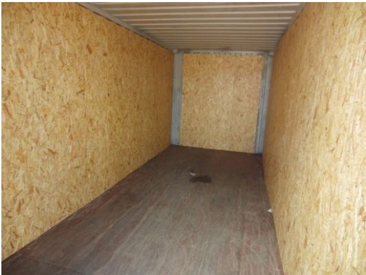
Figure 7.53 Lining a 40-foot container with chipboard panels
